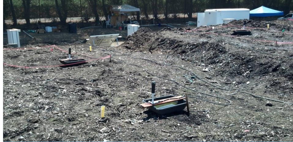
Solar Powered, Control Irrigated Aerated Static Pile
