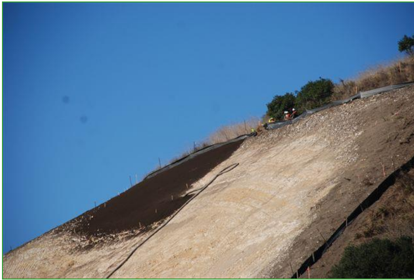
Main Street Materials – 1:1 slope, 4" compost Project near Lompoc
