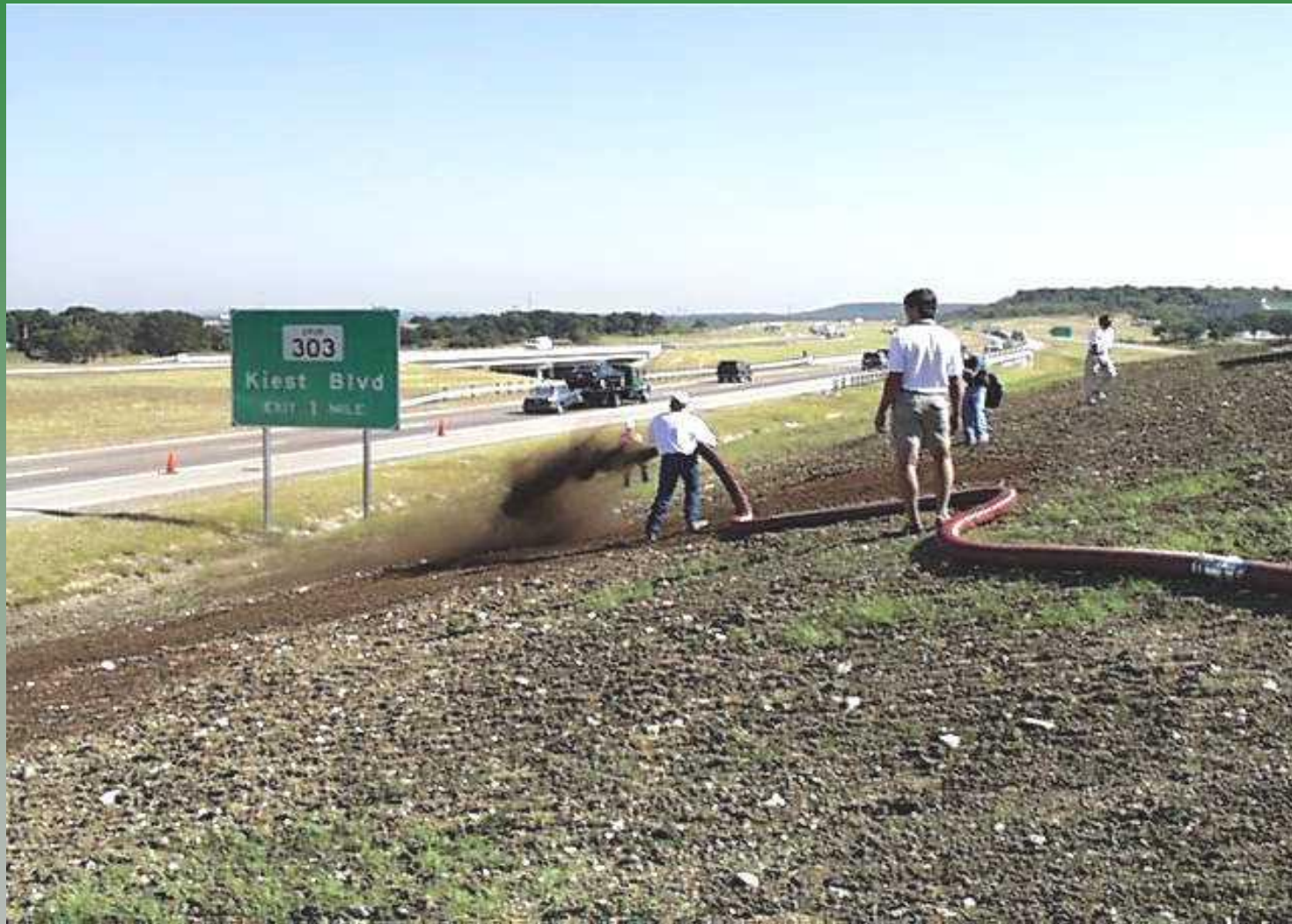
Dallas/Spur 408 Demonstration August 1999
