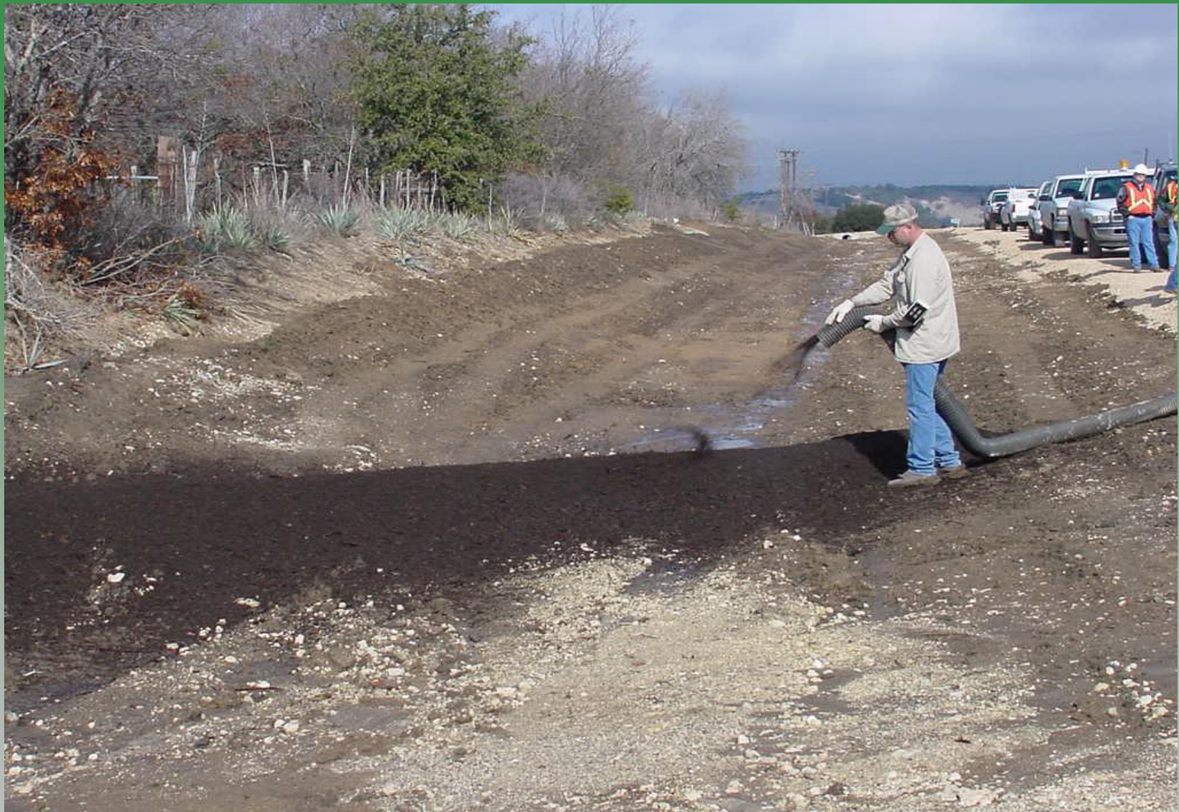
Compost Filter Berm Demonstration US HWY 281 Jan. 11th
