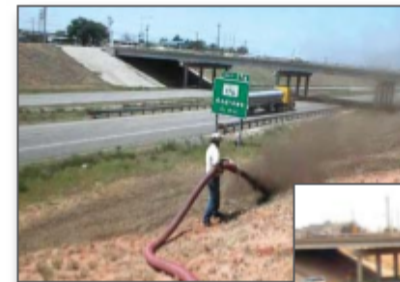
Figure 1. Applying a compost blanket on a bare and eroding slope
